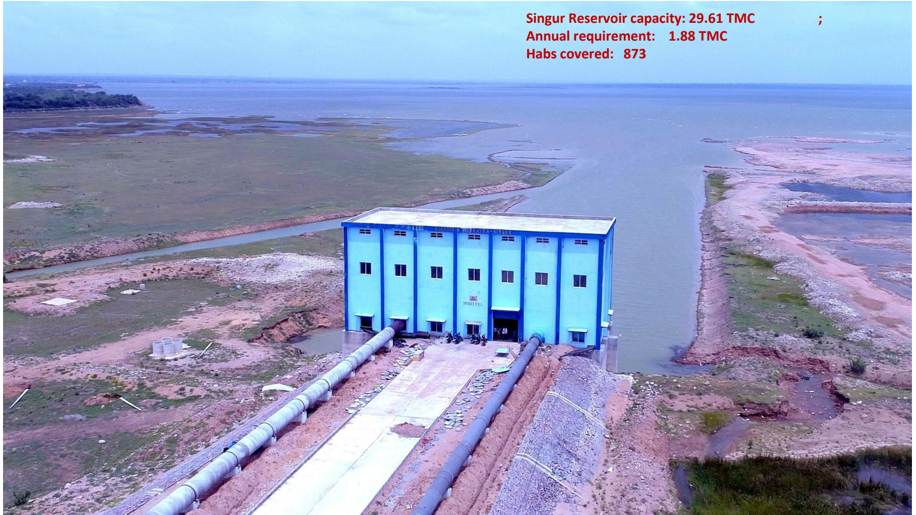
30m x 12m Intake well at Singur reservoir near Peddareddipet
