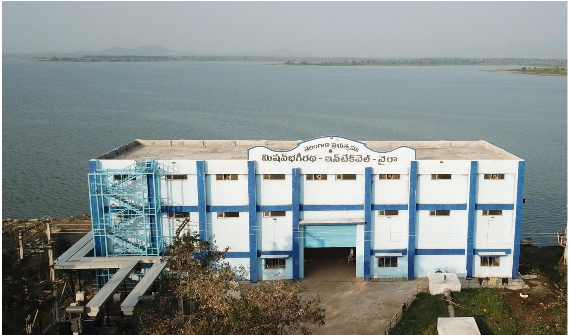
Intake well @ Wyra Reservoir
