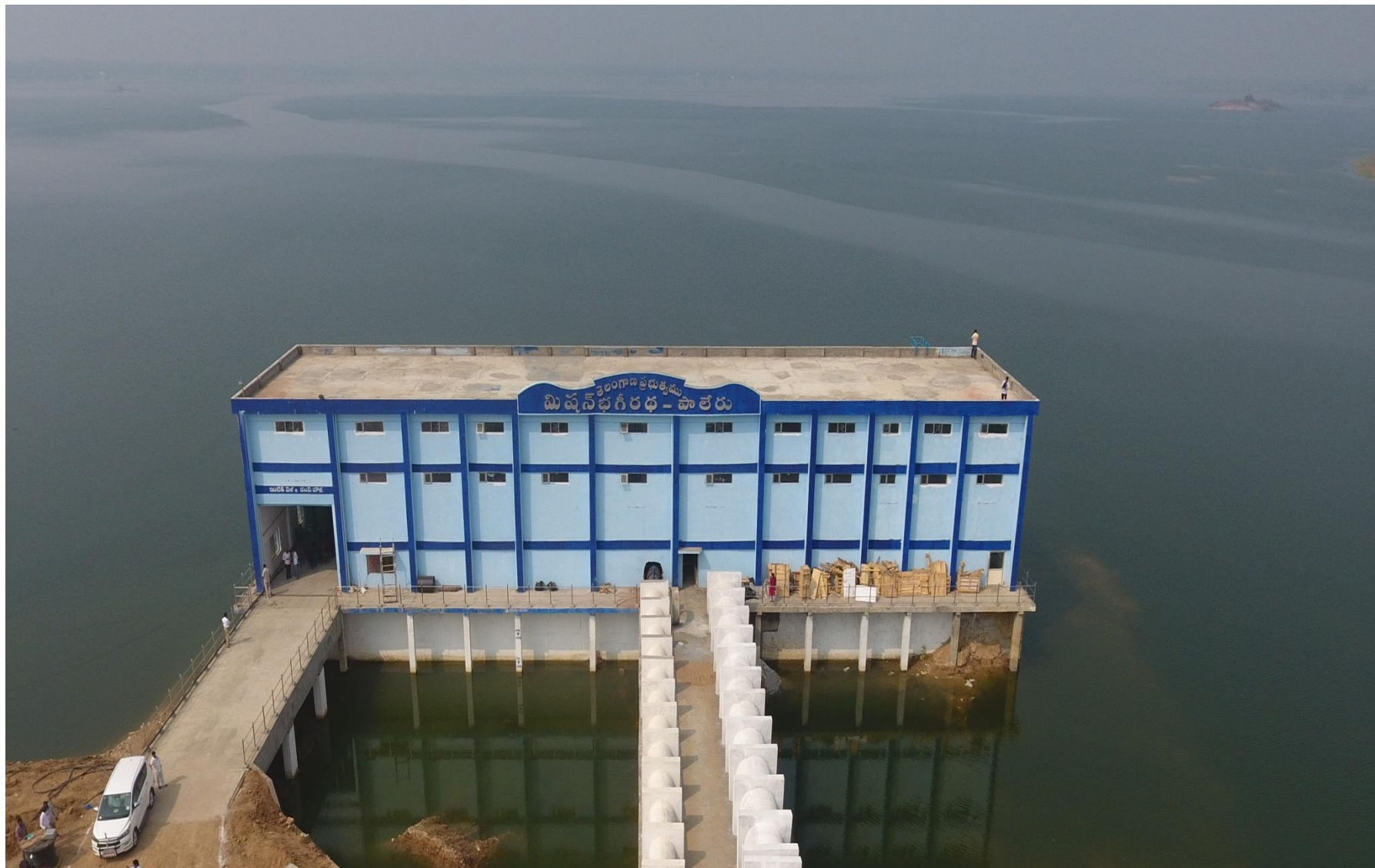
55m x 12m x 14m Intake well
